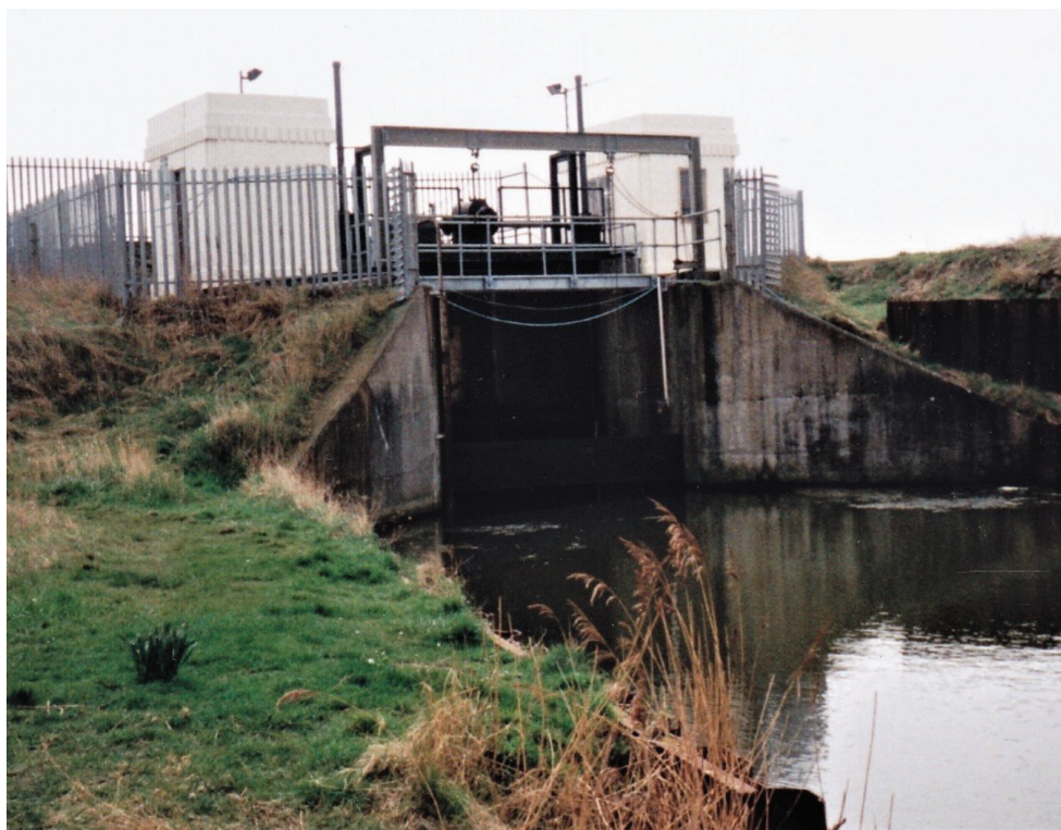
Roger Kennell (2000): The new sluice at Holland Haven built in 1937 to drain the Tendring Level, folRoger Kennell (2000): The new sluice at Holland Haven built in 1937 to drain the Tendring Level, following severe storm damage to the previous sluice.
